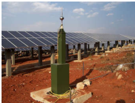
Fig.19. Yun nan shi lin Solar Farm telescopic mast
