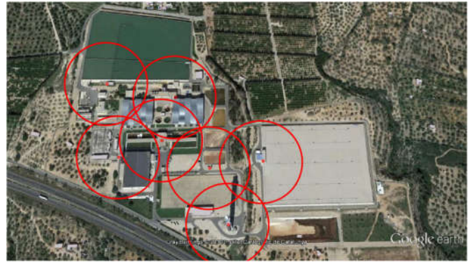
Fig.20. Consorci Aigües Tarragona, Water treatment plant
